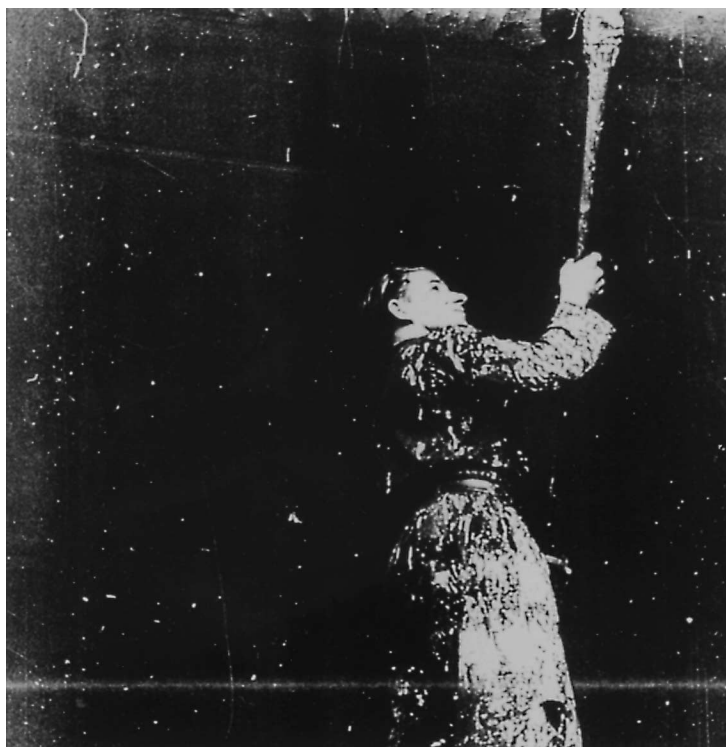
Fig. 3. Application of the ‘Doping’ compound.
